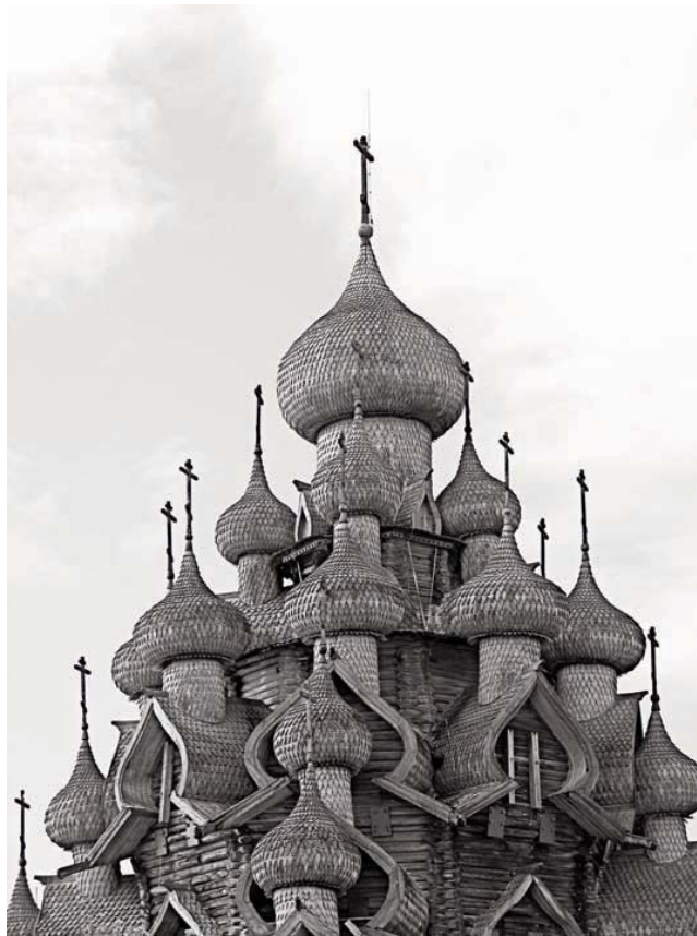
Preobrazhenskaya ( Transfiguration ), the onion-domed wooden church on the holy island of Kizhi, built in 1714 without a single nail
